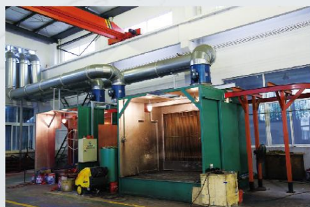
清洗喷漆设备 (Painting Equipment)
