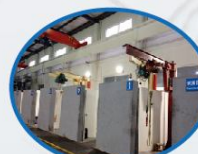
高压水密封、气密封试 (High Pressure Test)
